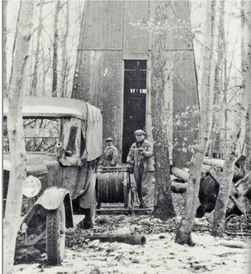
Figure 1. Logging survey at the Pechelbronn oil field (1928), Alsace, France. This is the same well in which Henri Doll, Roger Jost and Charles Scheibli, conducted the first electrical resistivity well logging operation in September, 1927. Source: Schlumberger.
