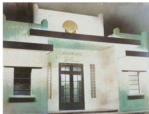
Figure 28. Front of the laboratory building of the Caribbean Petroleum Corporation in Maracaibo. It was the company's regional laboratory. Photo taken from Westermann, Tópicos Shell de Venezuela, 1941. Photograph colorized.
