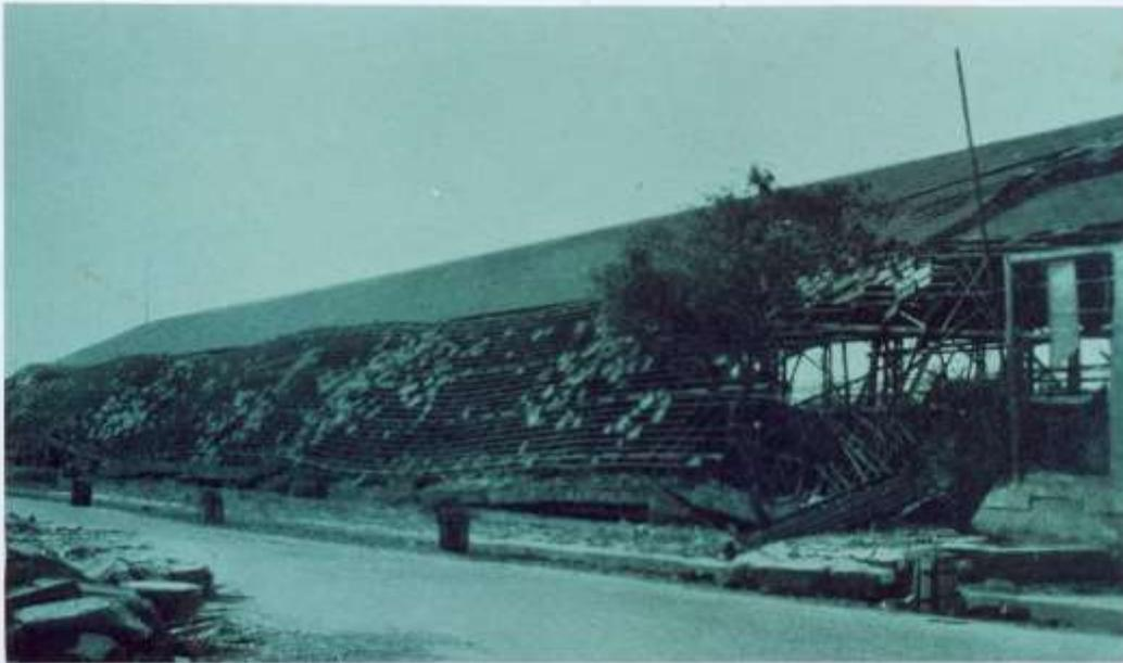
Fig. 5 Industrial de Manzanares, light steel structure. Central shed supported on steel posts was uninjured. Outer sheds supported on the outside by concrete wall were wrecked by collapse of walls.
