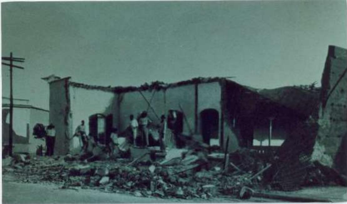
Fig. 12 Demolished concrete house; walls were of insufficient tensile strength.
