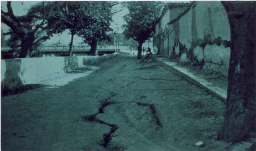
Fig. 7 Earthquake cracks in the alluvium bordering the River Manzanares
