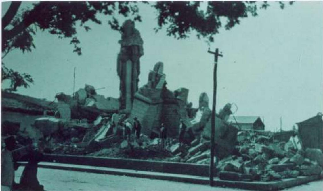
Fig. 13 Museum, heavy construction of poor mixture; very slight tensile strength; material can be crumbled in fingers.
