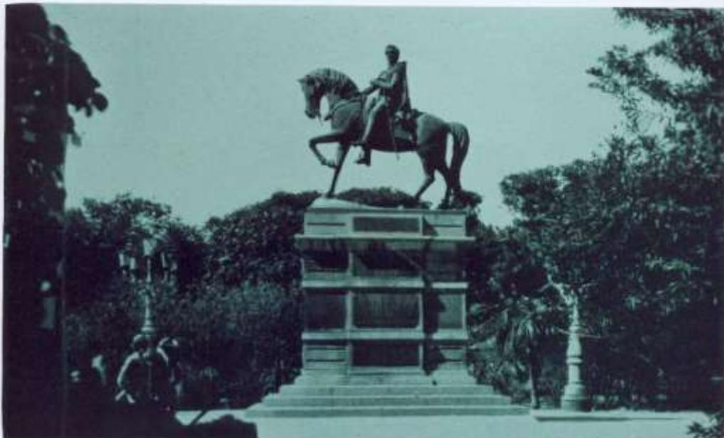
Fig. 11 Statue of Bolivar, uninjured; resting on stone and concrete foundation.
