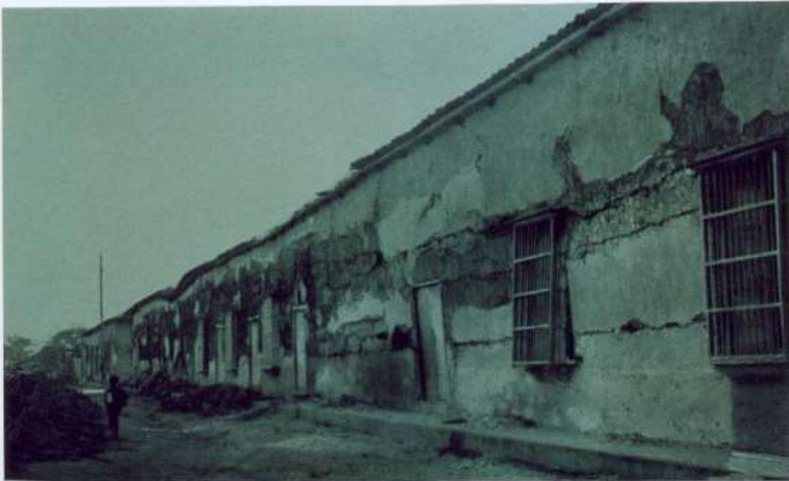
Fig. 14 Street in Cumana (calle Mariño); the interiors of these houses are wrecked by impaired walls and fallen roofs
