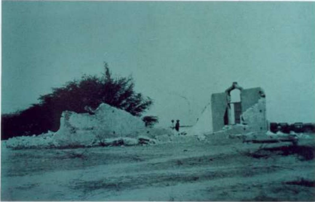
Fig. 4 Destroyed chapel at Caiguire. East-west wall at rear fell northward into the chapel
