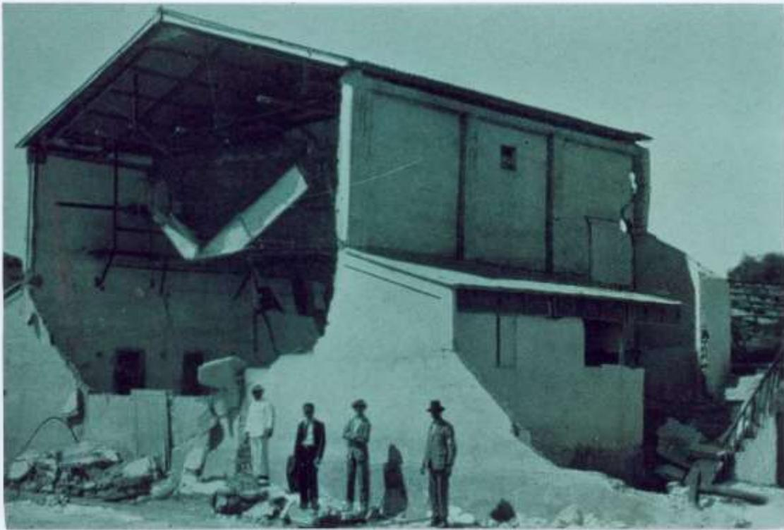
Fig. 19 Rear view of moving-picture theater. Rear wall fell northward and inward
