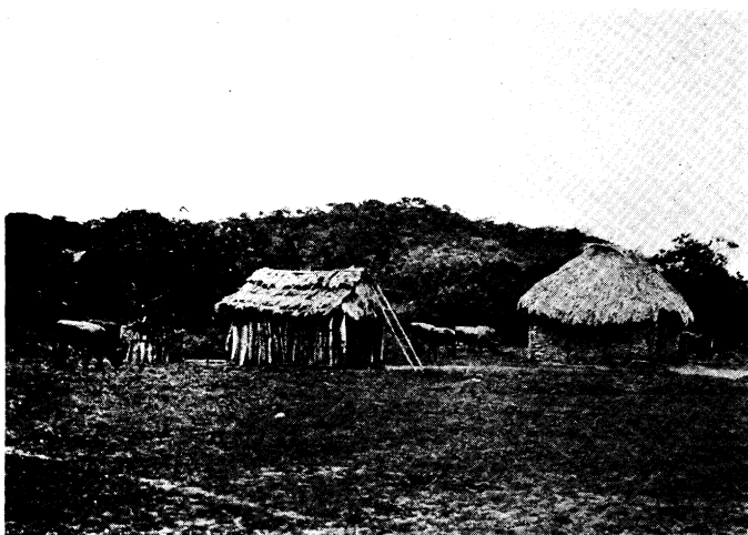
FIG. 9—Typical native houses near La Villa. The house on the right is made of intertwined boughs plastered with mud.
